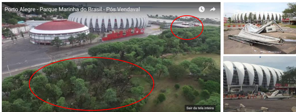
Figure 10. Full-scale damage to surroundings caused by downburst and no damage to stadium
