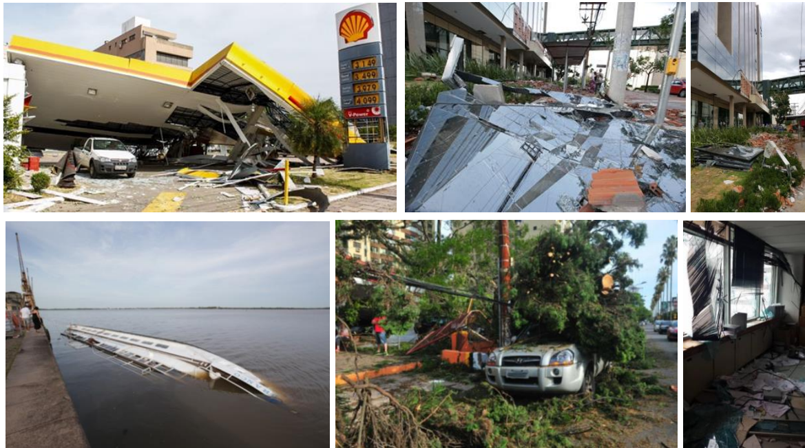
Figure 1. Examples of damages occurred during the Porto Alegre January 29, 2016, downburst event.
