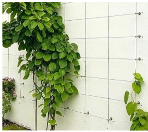
Fig. 8 Cables or wire net climbing system
