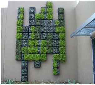
Fig. 3 Panel with soil substrate cells for planting
