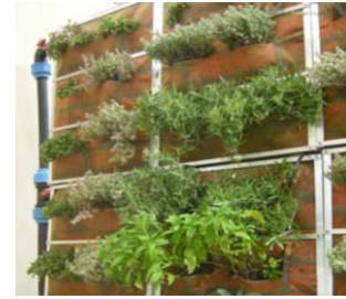
Fig. 5 Green wall with layer for cultivation
