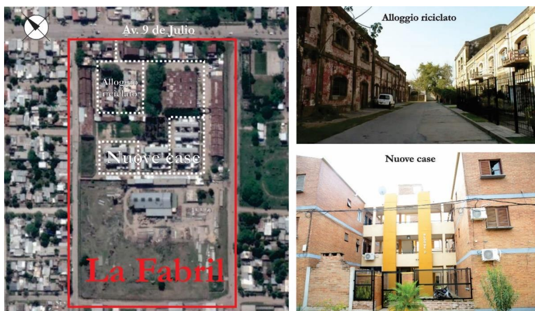
Figure 6 - Streets and housings (renovated buildings and new houses) nowadays at "La Fabril"
