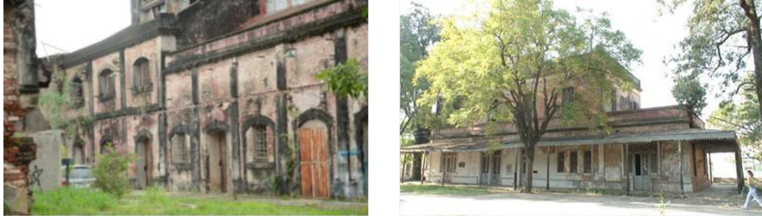
Figure 3 - "La Fabril" factory sheds: present state
