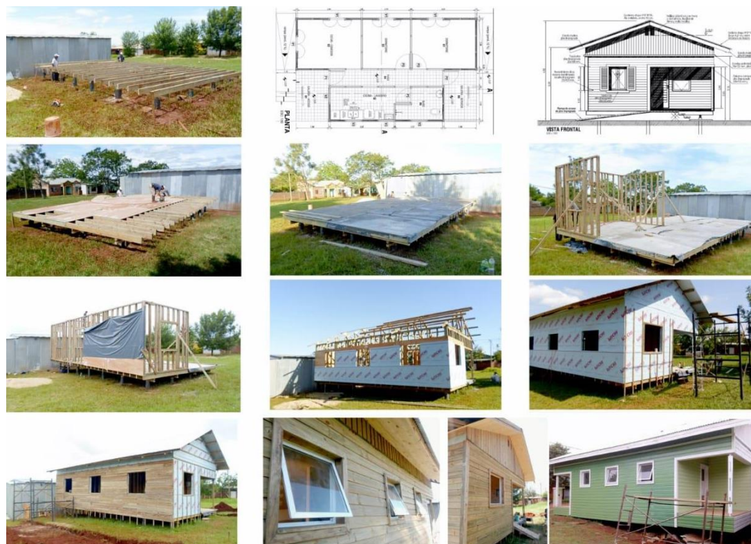
Figura 2. Floor plan, elevation and photographs of the construction phases of INVICO's viviendas sociales at the Virasoro locality. [© INVICO (drawings) and Erick Kennedy (photographs)]
