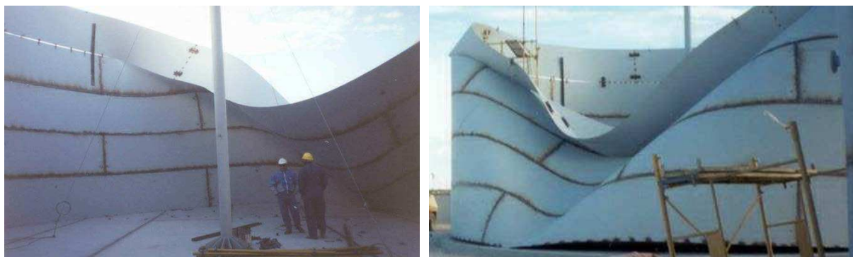
(a) (b) Figura 3: Tanque colapsado, (a) Vista interior, (b) Vista exterior.
