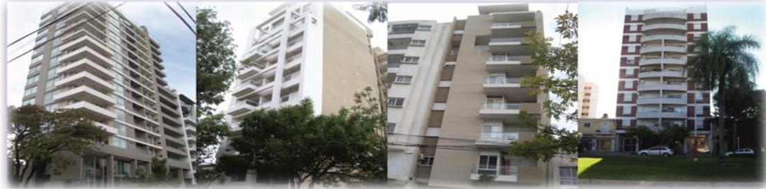
Figure 12: Image of towers in Resistencia densification area Source: Taken by author, 2013
